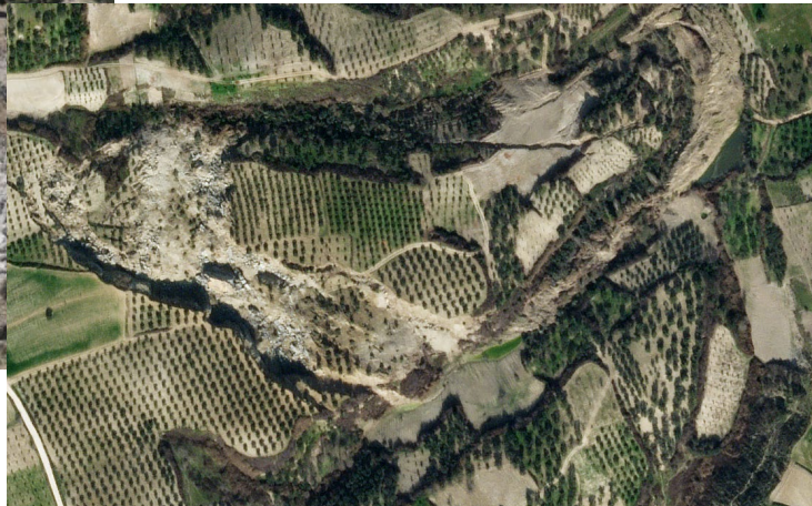
Tepehan landslide in satellite imagery [Image credit: Planet, SkySaf]
